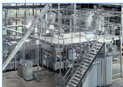
Supply and exhaust air system for an aseptic filling machine
