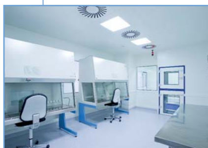
Clean room for cytostatics processing
